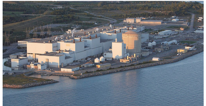
Darlington nuclear facility (Source: Public domain image by Ontario Power Generation via Wikimedia Commons).
