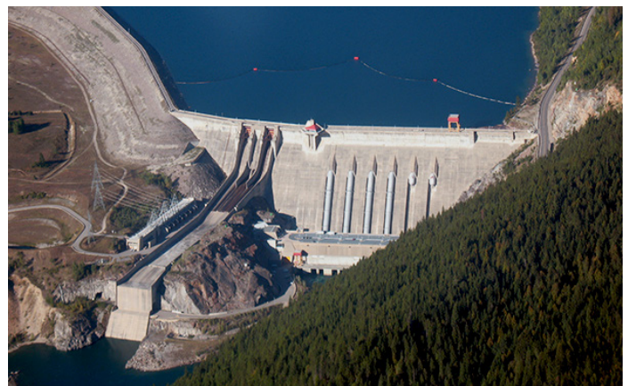
Aerial view of the Revelstoke Dam in Revelstoke, British Columbia. The blue at the top of the image is the reservoir (Source: Kelownian Pilot [CC BY-SA 3.0] recoloured via Wikimedia Commons).
